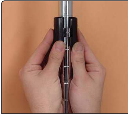
1. Snap plastic sleeve around post.
